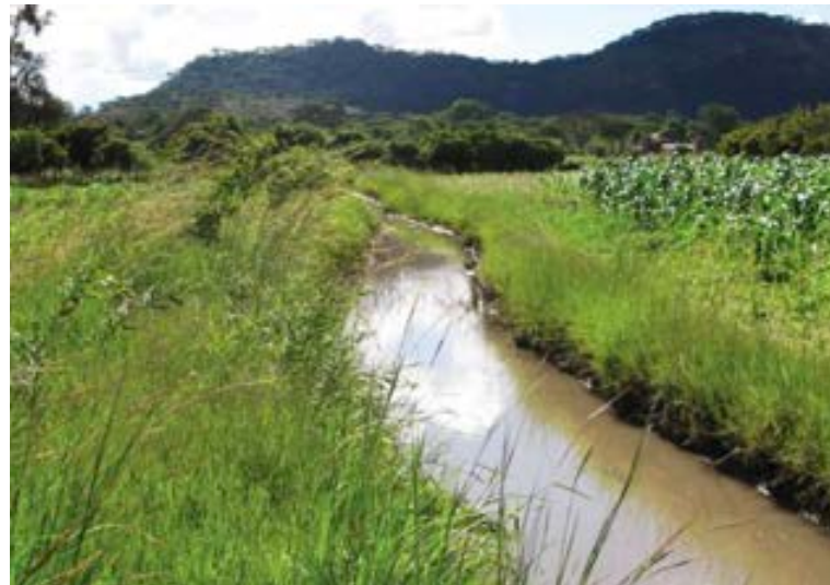
Caption: A swale collecting rainwater so that it sinks into the ground Credit: WSA
